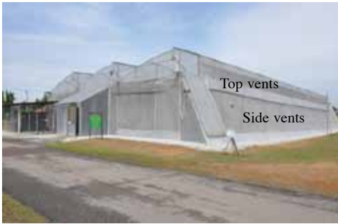
Plate 1. Controlled environmental structures at MARDI Headquarters, Serdang. The structures are covered with 200-micron transparent polyethylene and 50 mesh insect-proof netting. Top and side vents are part of natural ventilation system
