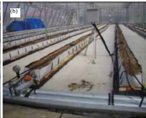
Plate 3. (a) Two rows of 25 mm diameter stainless steel pipe used in root zone cooling. (b) Pipe network and solenoid valves installed for root zone cooling
